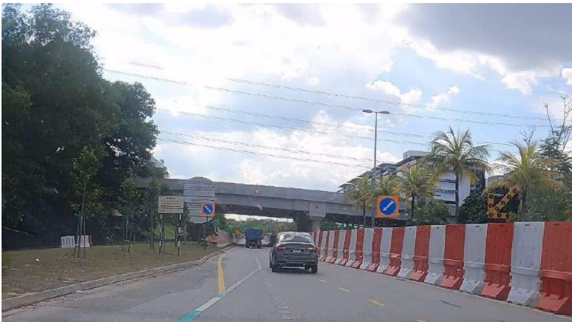
Figure A.6: Route B road conditions in Cyberjaya.
